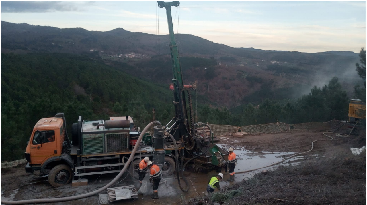
Figure 1. Drilling underway at Reservatório
